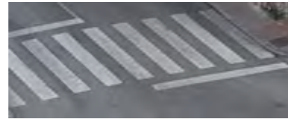
Fig. 2. Example of zebra crossing.
